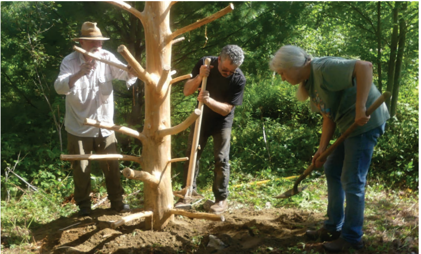
Geo Atwood, Dave Doherty and Carol Bennatti install a climbing tree in Popple Grove
