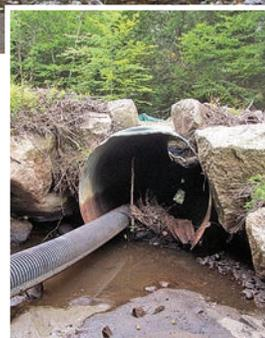
The Baker Brook culvert on the Valley Road suffered a complete wash-out in 2015 (shown after a temporary repair at right). This fall the damaged crossing was one of three replaced by cast-concrete bridges (above).
